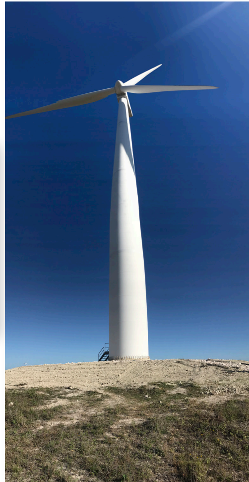
Adequately protecting the tower footings from erosion is vital.
