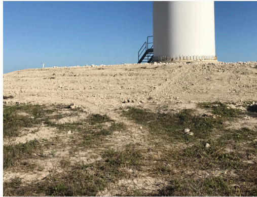
0.5% organic matter content in footing soil required a Biotic Soil Amendment be used to achieve desired vegetation results.
